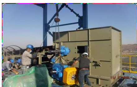
Belt conveyor 335CV05 - drive unit installation
